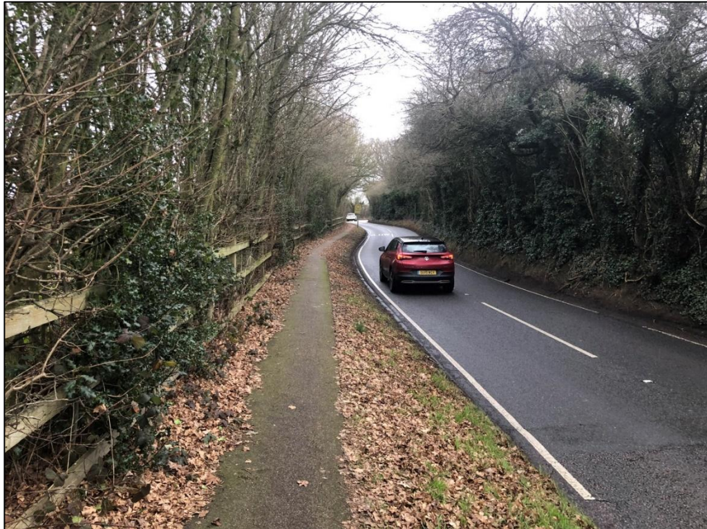
Image 3.2: Ascots Lane Footway
